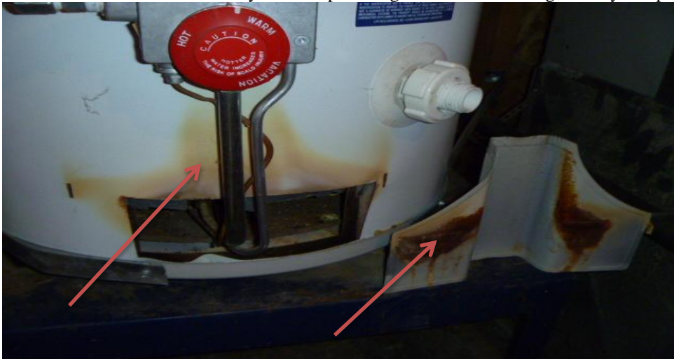
Figure 8 Flame roll-out scorching
