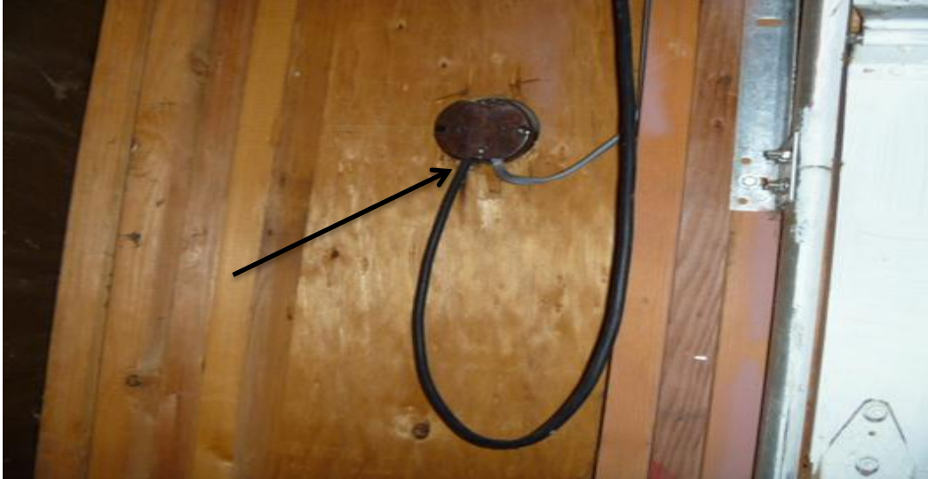
Figure 7 Non-Standard wiring
