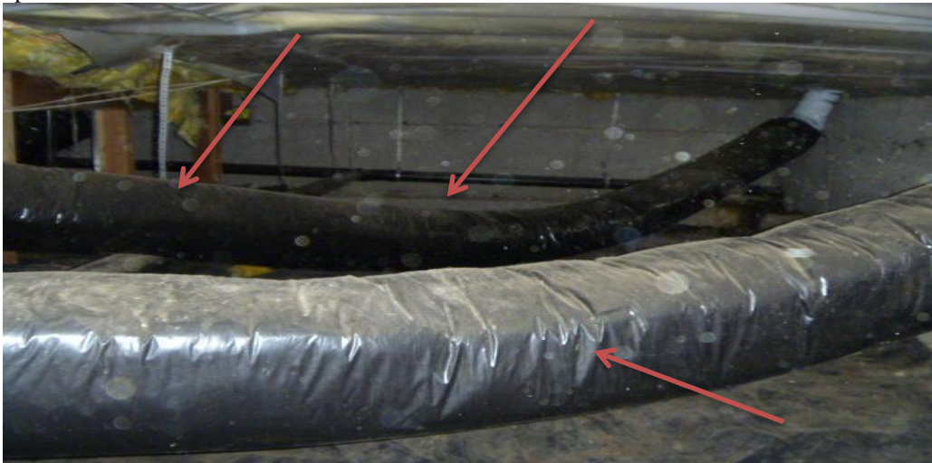
Figure 3 Unsecured ductwork
