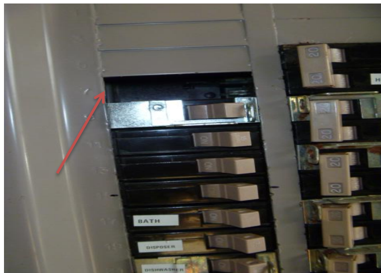
Figure 6 Missing "knock-out"
